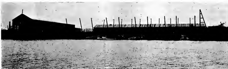
General View of the Albina Engine and Machine Works Shipyards.
